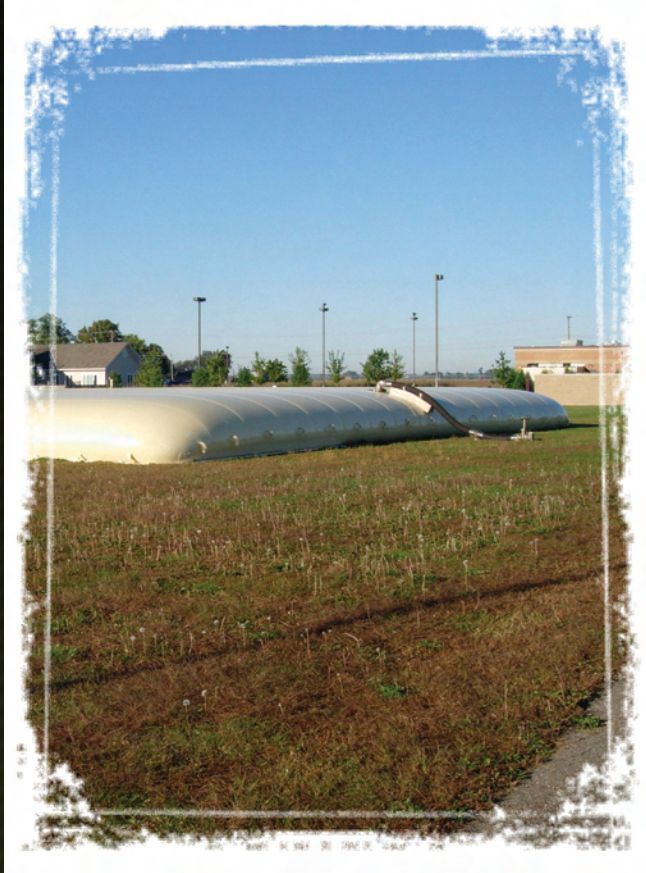
Shelter-Rite® Fuel Tank Farm Craney Island
